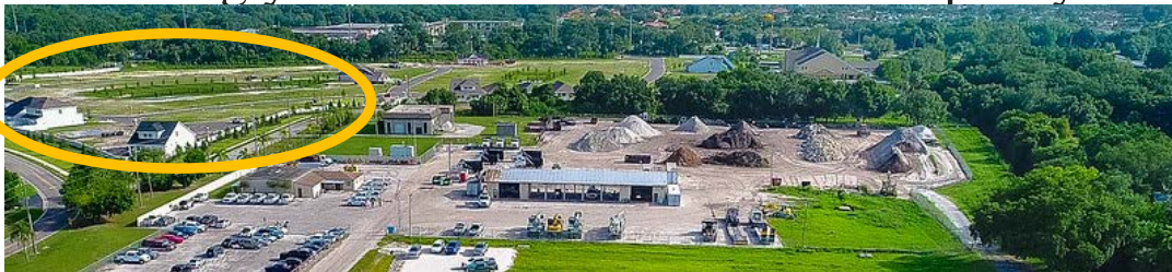
Stormwater Maintenance Yard
